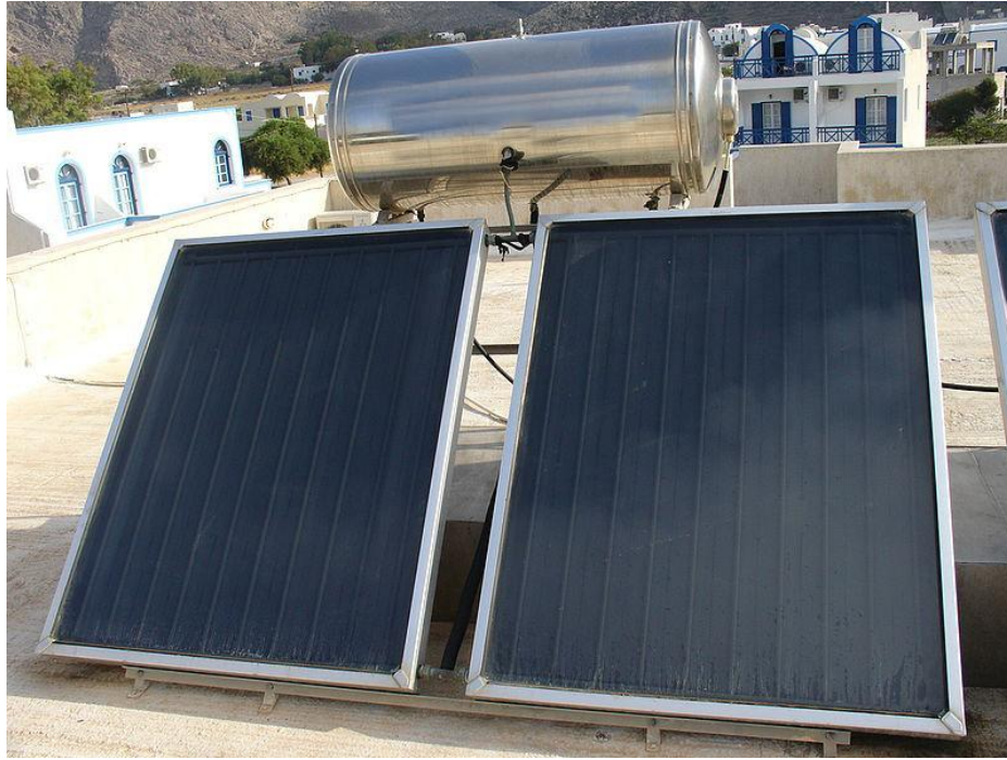
Figure 4.8. Flat plate solar thermal collectors used for heating water deployed on the roof of a hotel in Santorini, Greece (Credit: 23x2 from commons.wikimedia.org).
