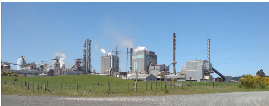
Figure 4.20. Kinleith Mill, a paper and pulp mill in Waikato, New Zealand. The building at the right is a cogeneration (produces both heat and electricity) power plant burning wood waste. The energy is then used to power paper production. (credit: Ingolfson).
