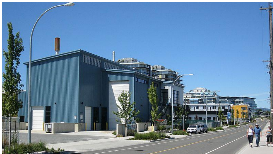
Figure 4.21. Biomass gasification plant at the Dockside Green community in Victoria, British Columbia, Canada. This operation converts wood waste into methane gas that can be used for heating and hot water (credit: John Newcomb).
