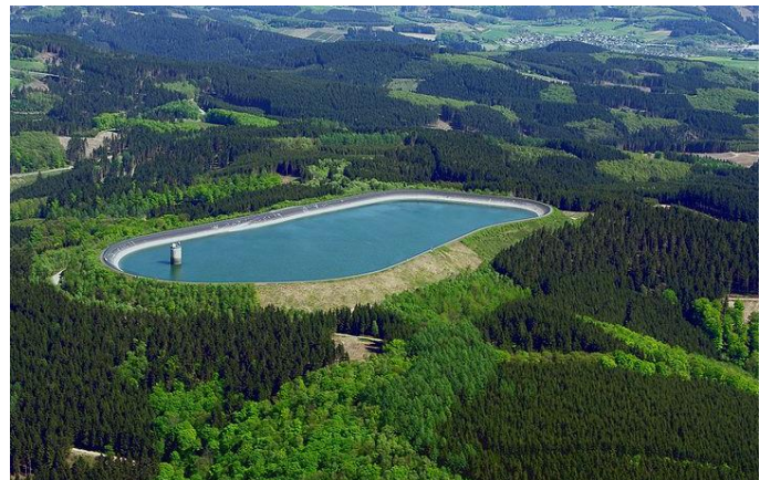
Figure 4.14. Upper basin of a pumped-storage facility in Rönkhausen, Germany (credit: Dr. G. Schmitz).
