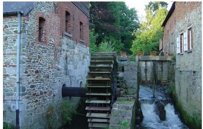
Figure 4.11. Traditional water mill dating from the twelfth century in Braine-le-Château, Belgium. Note that the mill itself is not in operation at the time this picture was taken. When operating, water will move the slats of the mill, causing the rotor to turn, and providing power for machinery inside the building. Credit: Pierre79, from Wikimedia commons
